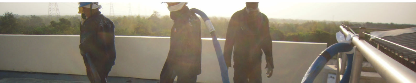
Nestle Pasuruan Roof Deck
