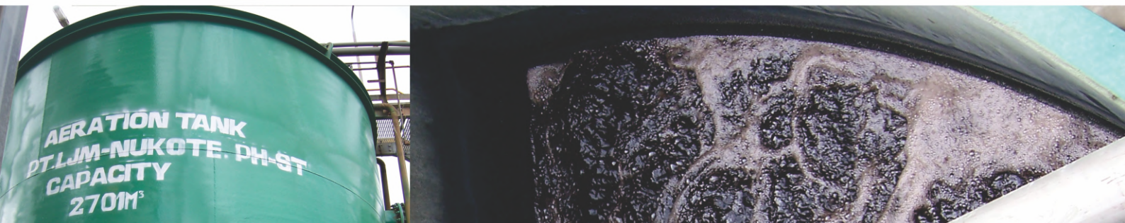
Waste Water Tank
