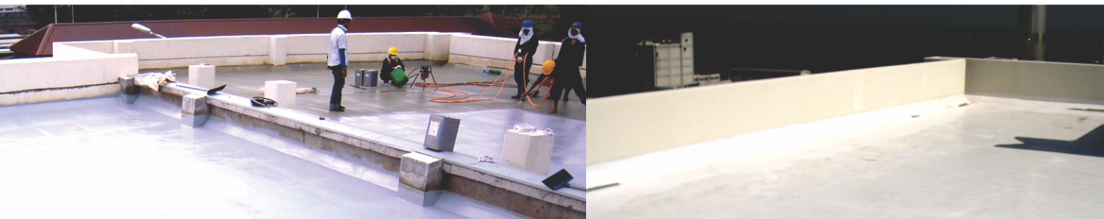
Nestle Ckd roof deck
